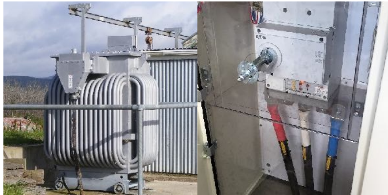
Figure 1: The network-consumer boundary between a distribution transformer and the main switchboard (MSB) of a regional council pumping station
